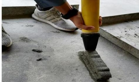
**Figure 3: Manual extrusion process using manual cement pump**
