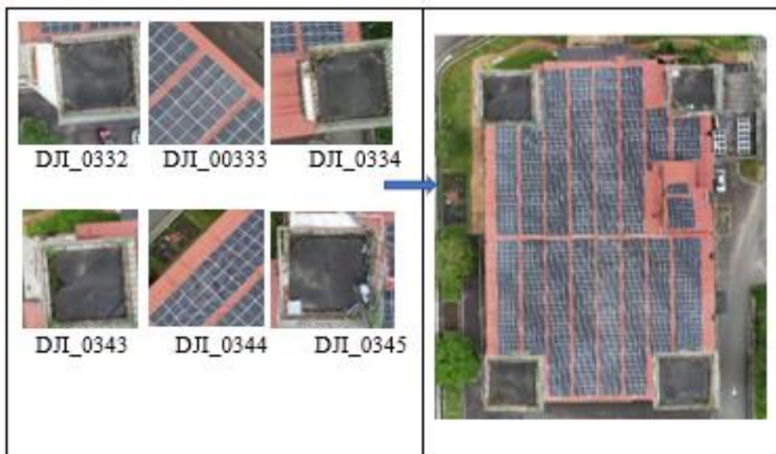
Figure 4: Steps of image processing F2 examination hall UTHM
