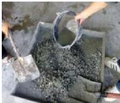
Figure 2: Process of batching and mixing the materials
