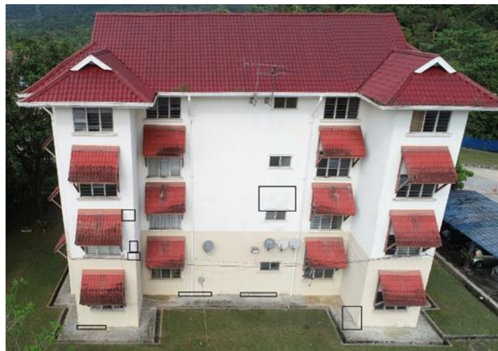
Figure 8: Rear elevation of Kuaters Kediaman INSTUN
