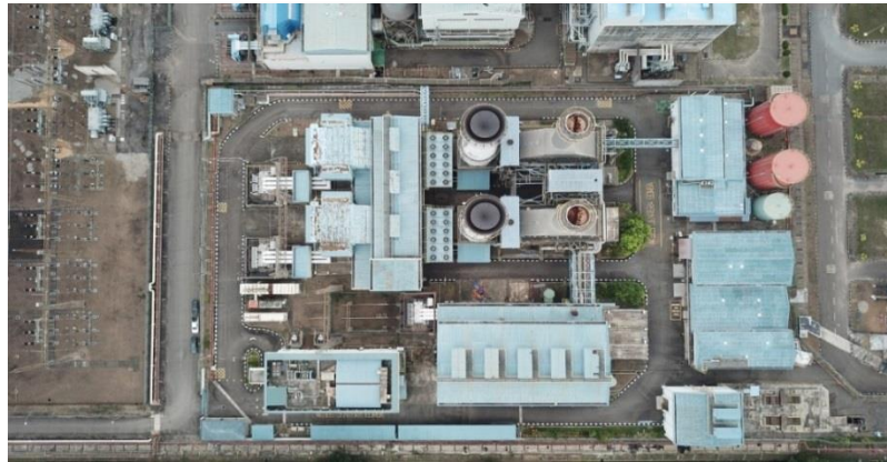
Figure 3: Location of site visit project for demolition work
