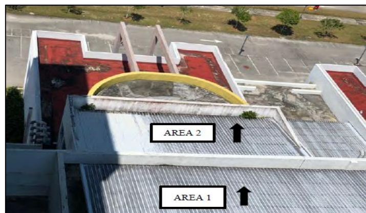
Figure 1: The catchment area at Geotechnical Lab, UTHM [17]
