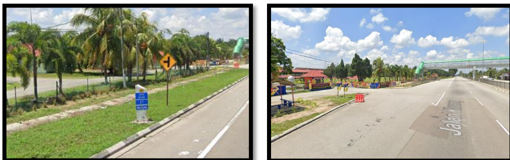
Figure 4: Signage and Road Facilities at Sekolah Menengah Kebangsaan Seri Gading
