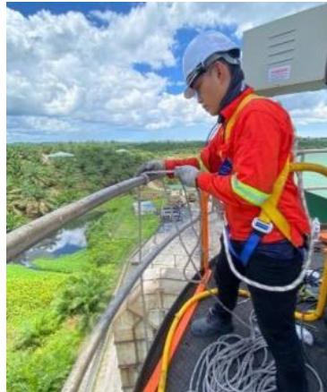
Figure 1: Workers lifting load manually
