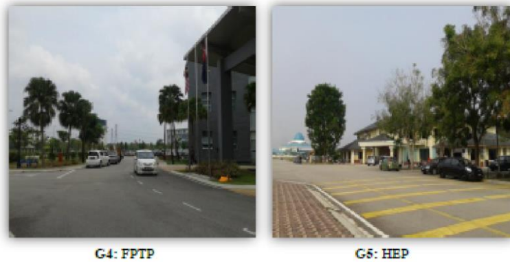
Figure 5: Photo of existing condition – building area (Author, 2014)
