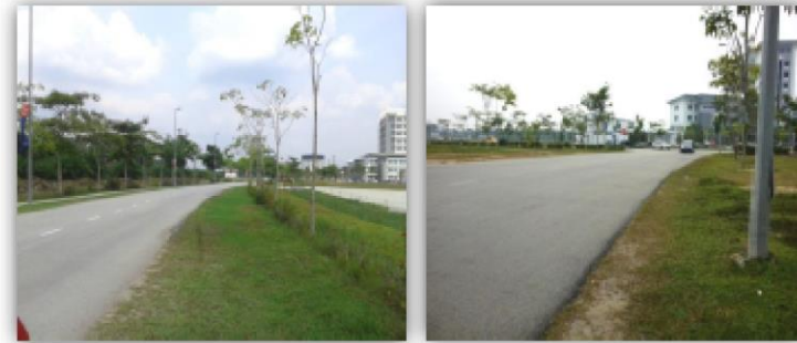
Figure 3: Photo of existing condition – roadsides
