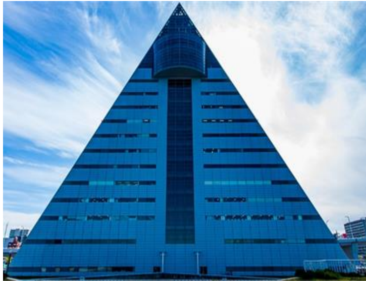
Figure 1: ASPAM building (Chris, 2017)
