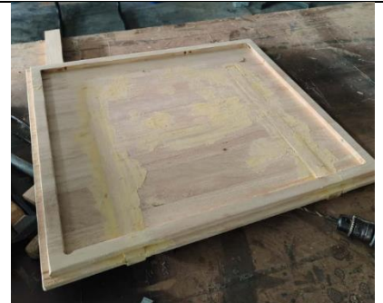
Fig. 27 Process Applying Wood Filler on Defects Area
