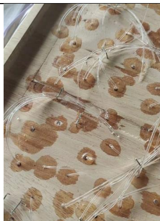
Fig. 17 Process Fastened Optical Fibre on Panel Using Staple Gun
