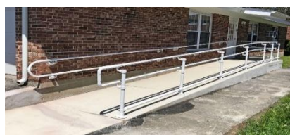
Rajah 2: Contoh susur tangan (Simplified building, 2020)
