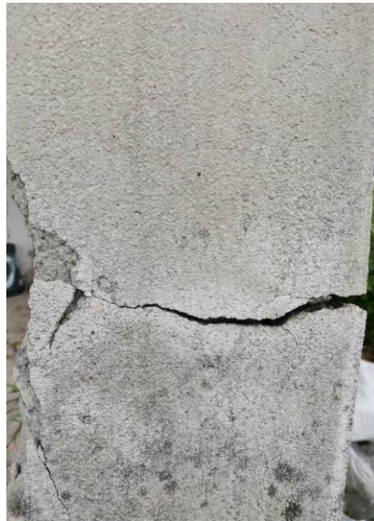
Figure 1: Crack on the column found at the car porch
