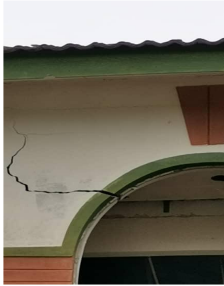
Figure 4: Cracks found above the window
