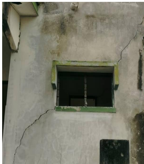
Figure 8: Cracks found on above and below the window
