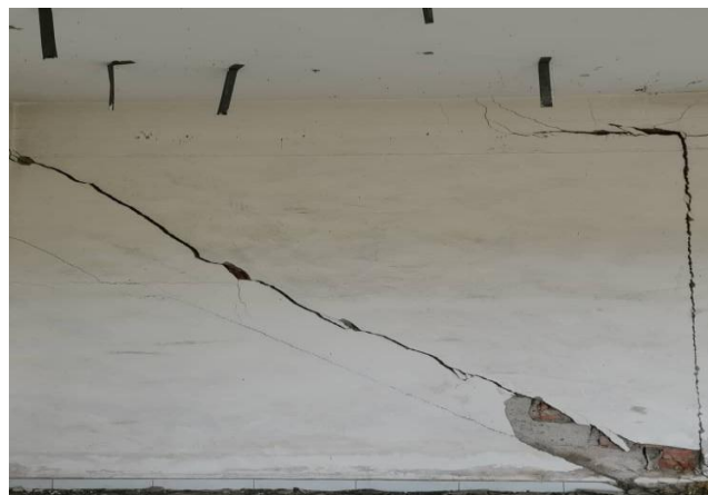
Figure 3: Crack on the wall found at the living hall
