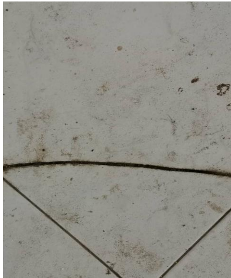
Figure 7: Cracks found on the floor
