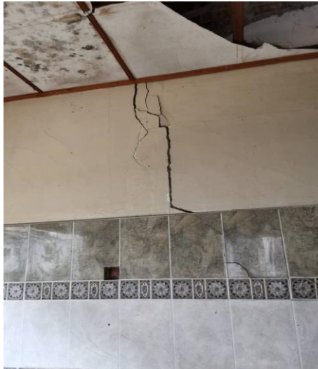
Figure 5: Cracks found on the finishing wall
