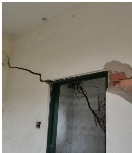
Figure 6 Cracks found above the door
