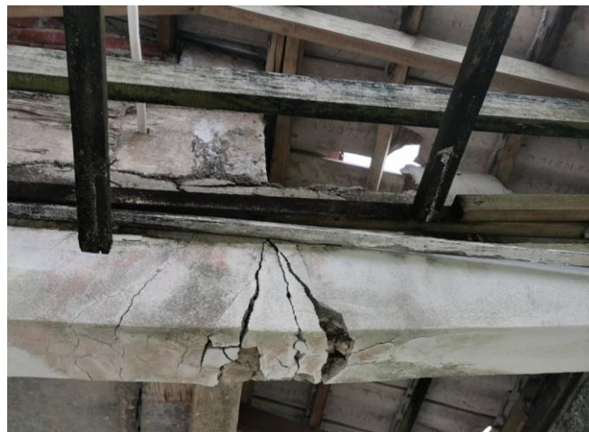
Figure 2: Cracks on the beam found at the car porch
