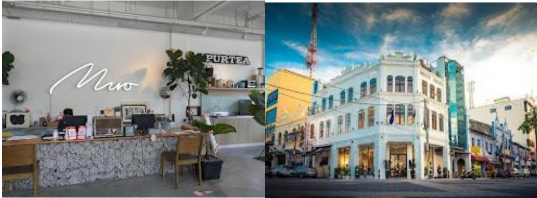
Figure 5: Building of Muo Boutique Hotel that has been renovated
