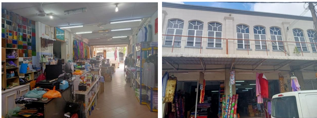
Figure 7: Building of Mubarak & Family Trading that has been renovated
