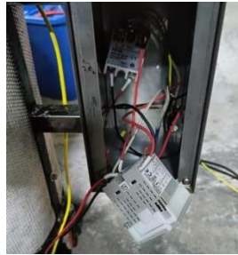
Figure 4: Control unit installation
