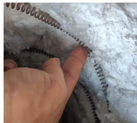
Figure 5: Installation of heating element
