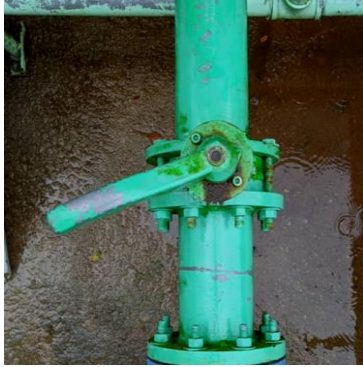
Figure 5: Butterfly valve (V101) before maintenance
