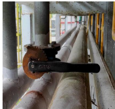
Figure 8: Butterfly valve (V201) after maintenance
