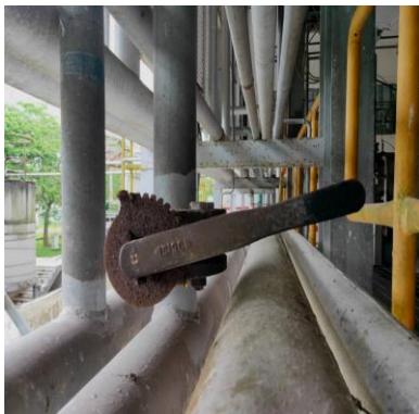
Figure 7: Butterfly Valve (V201) before maintenance
