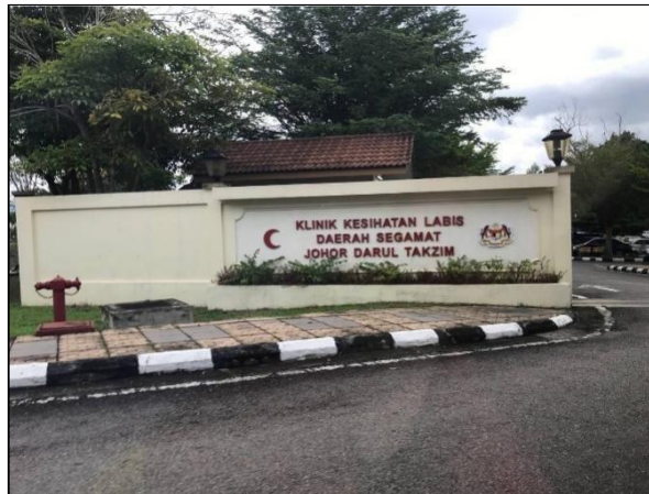
Figure 1: One of the Klinik Kesihatan for preliminary inspection
