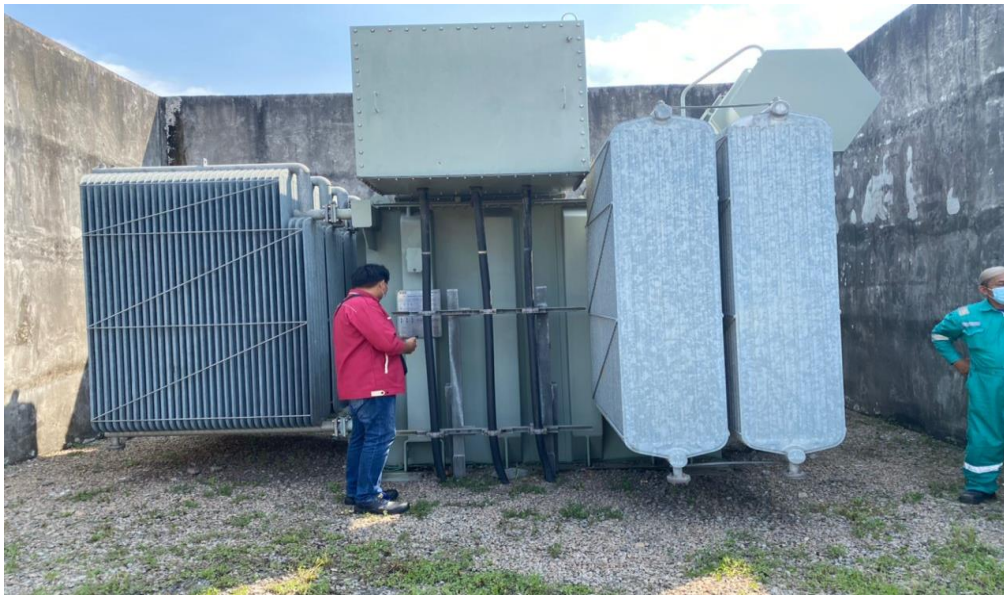
Figure 1: Transformer 66kv/470V
