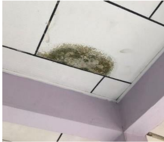
Figure 1: Mould Growth
