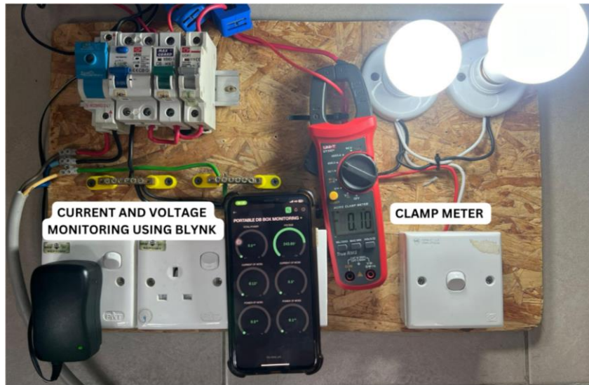
Fig. 7 Current Transformer SCT-013 Sensor Testing
