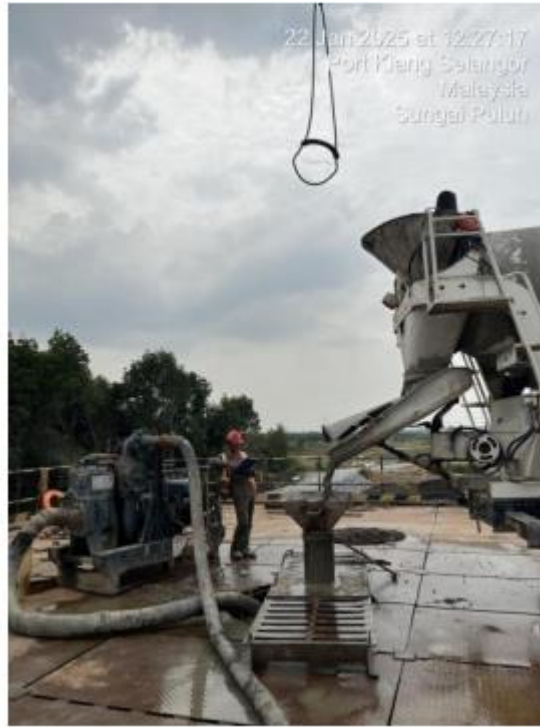
Fig.5: site personnel recording every drilling rig work phases
