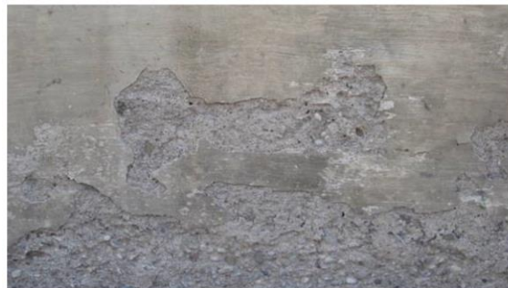
Fig. 1: Effect on the concrete surface when a release agent is not applied (Qian Jiang et al, 2023).
