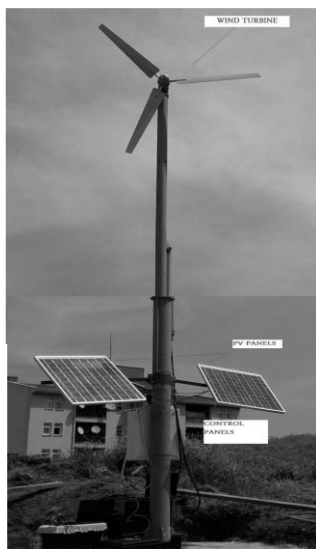
Fig 1 A picture of the constructed hybrid system
