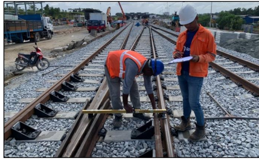
Fig. 4 Measuring checkrail flange way gap
