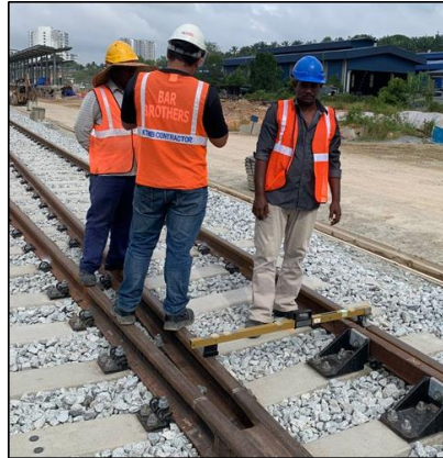
Fig. 2 Measuring track gauge at turnout
