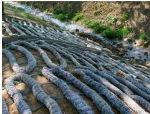
Figure 2.1: Geotextiles on Slope Surface [4]
