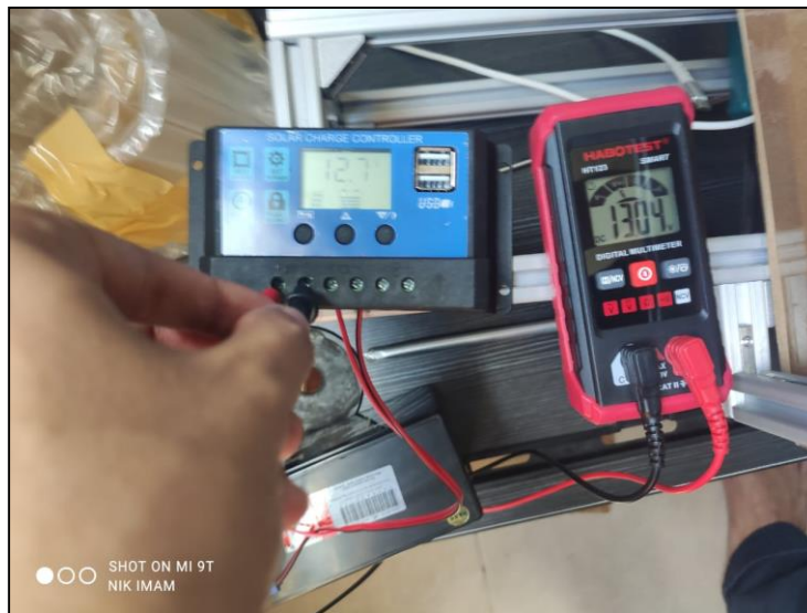
Fig. 6: Measuring Voltage With Multimeter
