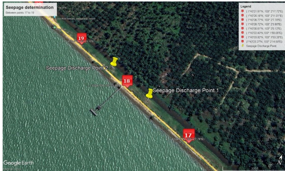
Figure 5: 2 Points are selected based on the severity of seepage
