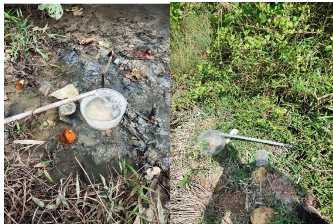
Figure 2.3: Severe seepage point current situation on point 1 and point 2.
