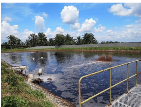
Figure 1: Palm oil mill effluent pond
