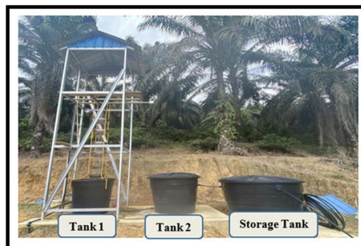
Figure 4 : Arrangement of Sand Filtration water tank
