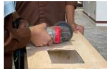
(c) Cutting opening for window
