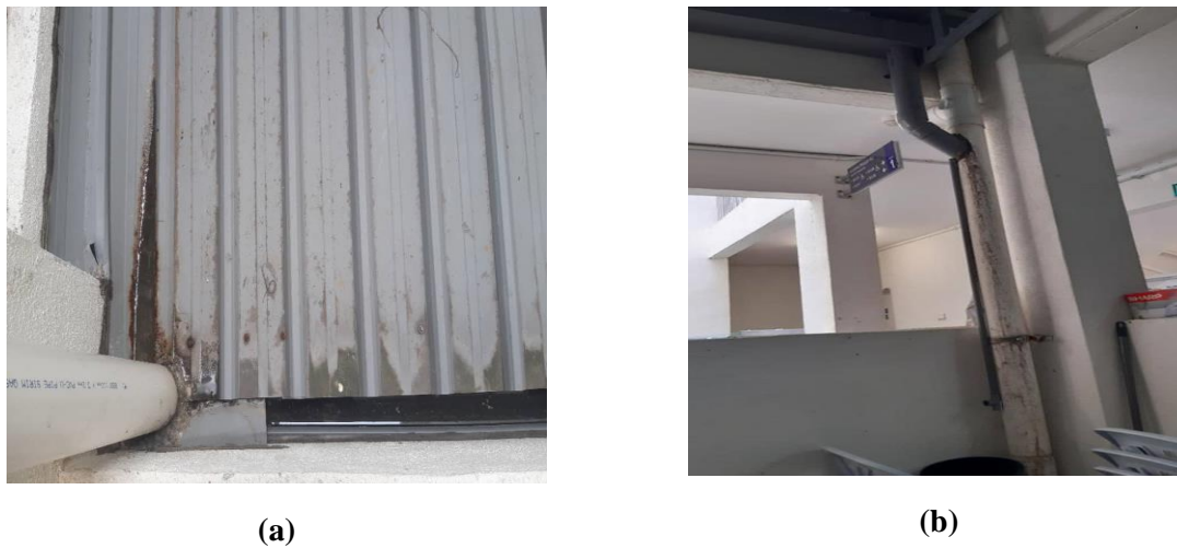
Figure 1: Study area (a) roofing condition (b) pipe connected to gutter
