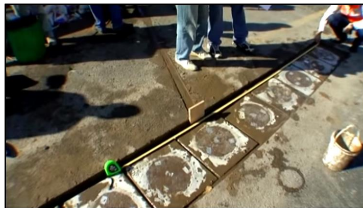
Figure 2: Installation of piezoelectric
