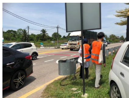
Fig. 7 No Proper Guardrails Extension
