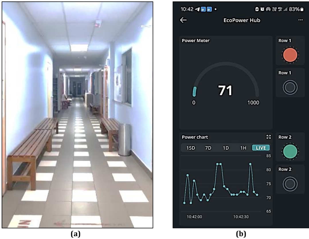
Fig.5 (a) Level 2 Corridor Lights Turned ON, (b) IoT Remote Dashboard
