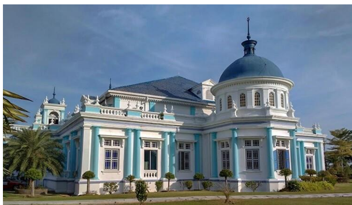
Fig. 1 Sultan Ibrahim Jamek Mosque
