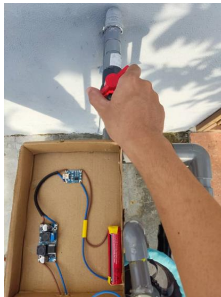
Figure 8: Adjusting valve of water flow control through Pico hydro generator module
