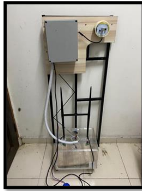
Fig. 5 Control panel Box
