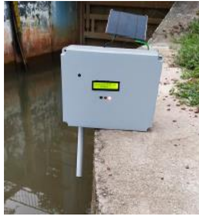
Fig. 9: Prototype placed at Pintu Air beside flood gauge
