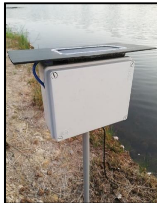
Figure 6: Installation of sensor node at Sungai Batu Pahat
