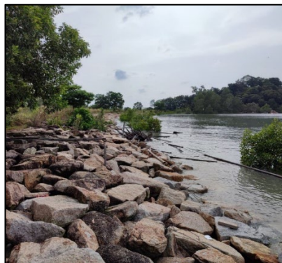
Figure 5.4: Rock revetment in Tanjung Laboh
