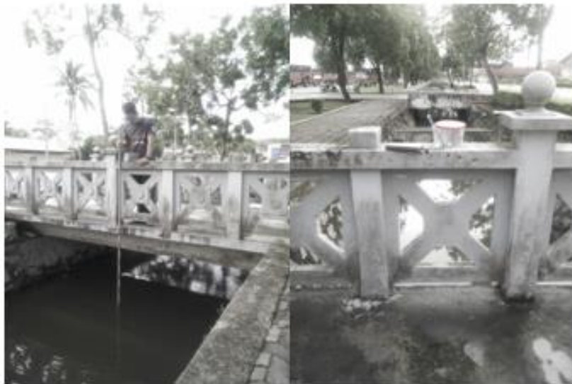
Fig. 4 - Actual experiment setup at the drain between block E14 & E15
