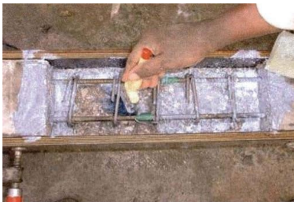
Fig. 2 Application of primer and repair material [10]
