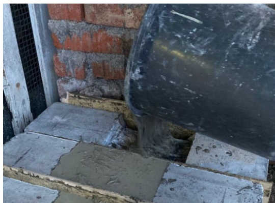
Fig. 6 Grouting mortar mix sample
