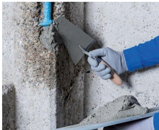
Fig. 1 Patch repair on concrete structure [9]
