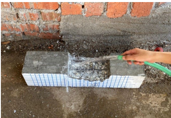
Fig. 4 Wash the defect area by water
