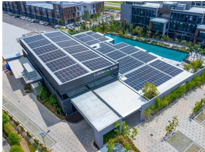
Fig. 18 Rooftop solar PV system (271.4 kWp)
