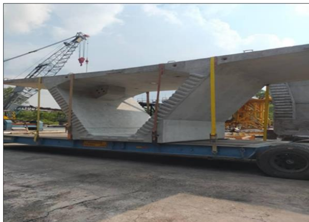
Fig. 2 Segmented box girder
