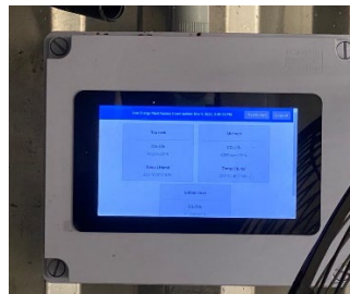
Fig. 4 - LEPF system display attached next to the racks
