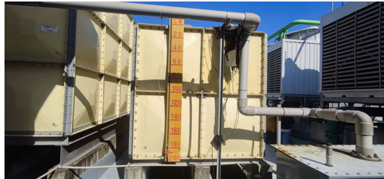
Fig. 5 - Depth of RWH storage tank
