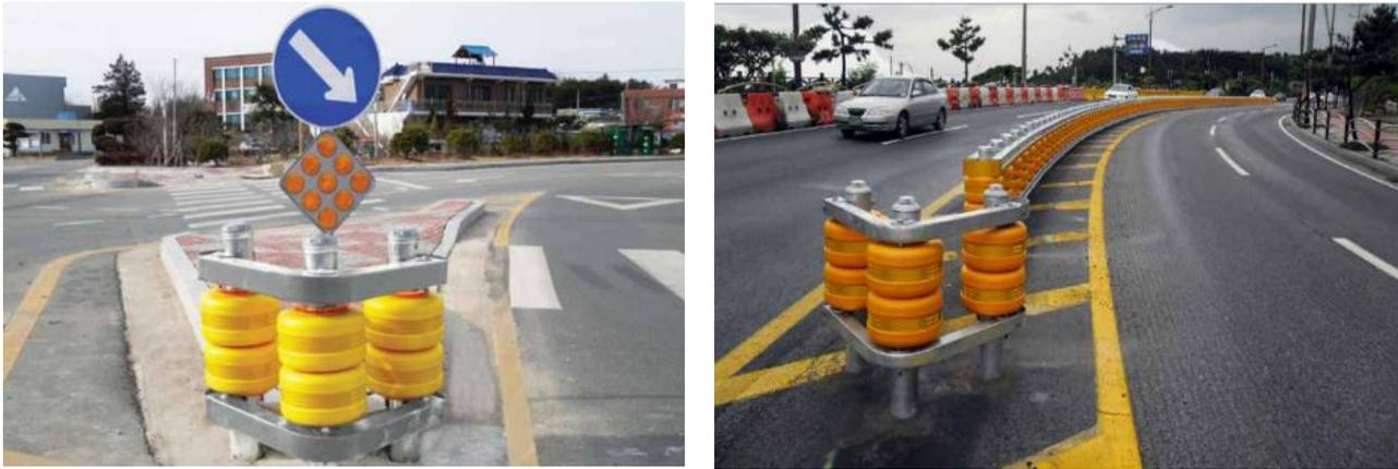
Fig. 5 - Median rolling barrier [11]
