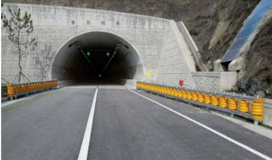
**Fig. 2 - Roadside rolling barriers at straight road [13]**
