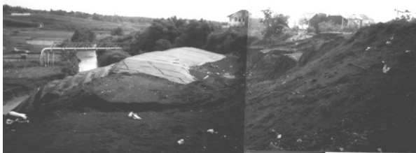
Fig. 34 View of the slope failures from the river (photographic documentation, Rahardjo).
