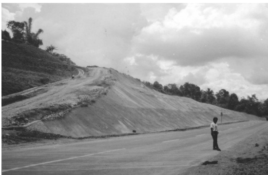
Fig. 10 Protection of the cut slope from severe weathering located at Citatah, West Java (photographic documentation, Rahardjo).
