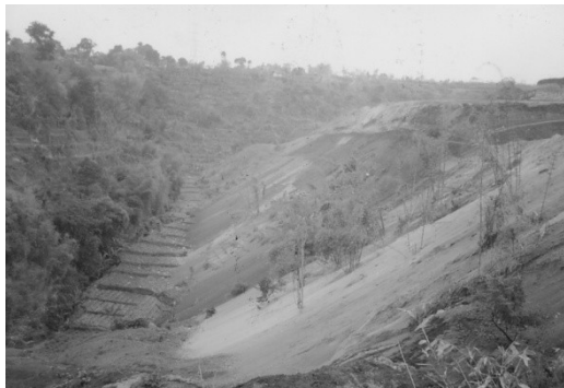
Fig. 17 Uncontrolled high fill embankment, North of Bandung (photographic documentation, Rahardjo).
