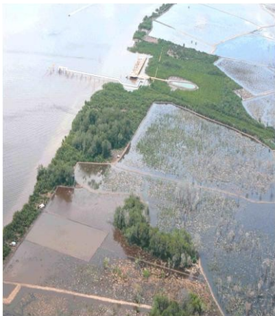
Fig. 9 Initial condition of the project site [20].
