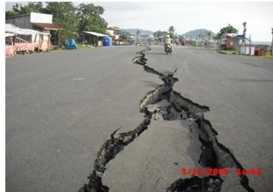
Fig. 27. Lateral displacement in Padang earthquake (photographic documentation, Rahardjo)
