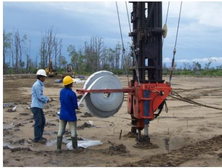
Fig. 8 Installation of the Vertical Drain (PVD) (photographic documentation, Rahardjo).
