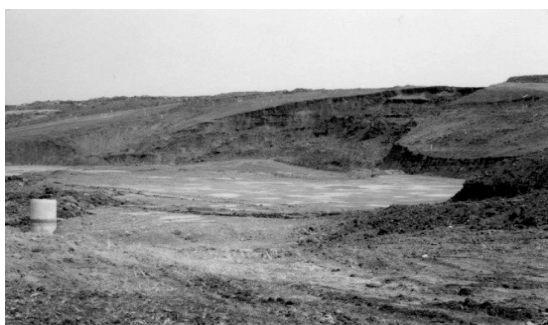
Fig. 22. Failures of slopes consisting of sand fill materials (photographic documentation, Rahardjo)
