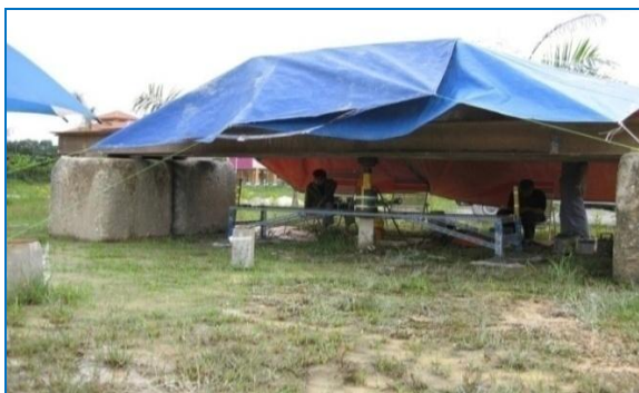
Figure 9: Full scale pile loading test was underway
