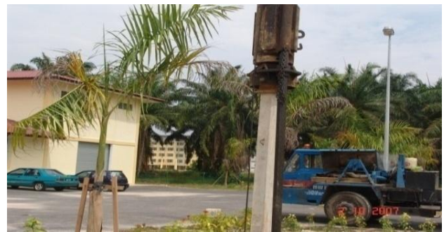
Figure 7: Pile being driven at research location
